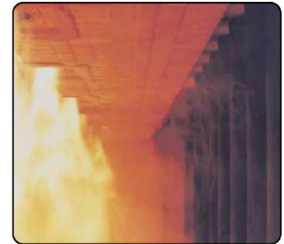
Tubes in a steam reformer
