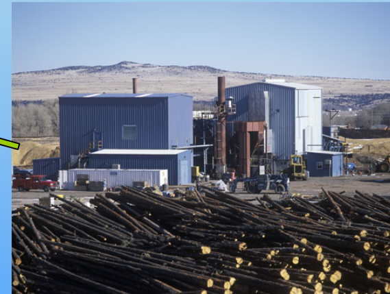
3 MW BIOMASS PLANT EAGAR, ARIZONA
